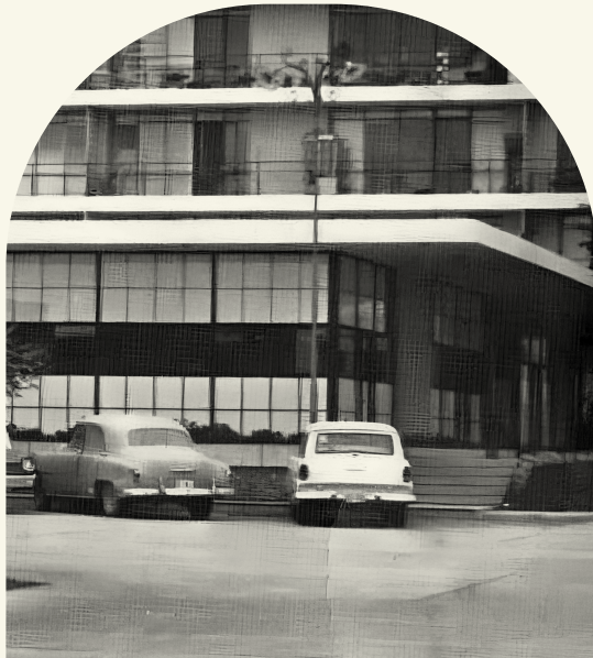
LA LINTERNA RESTAURANT, LA AURORA, 1960'S
